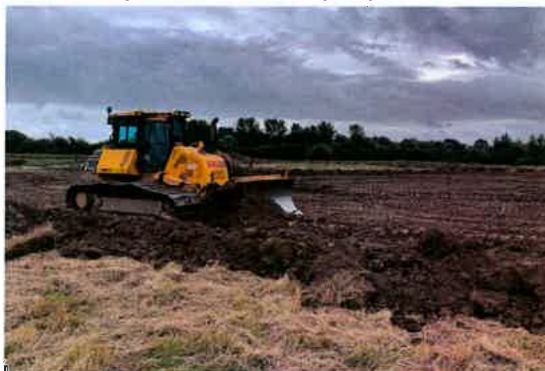
Bulldozer excavating the new 'scrape', October 2023.
